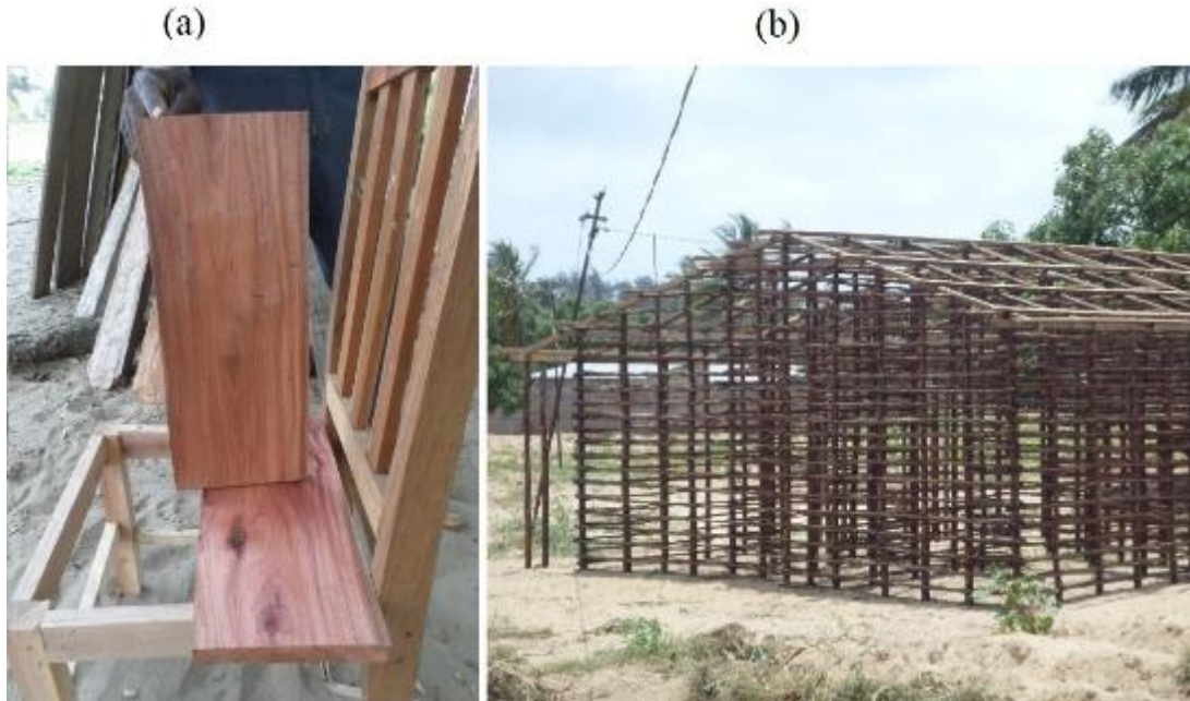
Figure 5.1. Mangrove wood usage: (a) a chair built with Xilocarpus granatum mangrove wood and (b) a house frame built with Ceriops tagal poles. (Bairro Farol, Chinde, Zambezi delta, October 2016).
