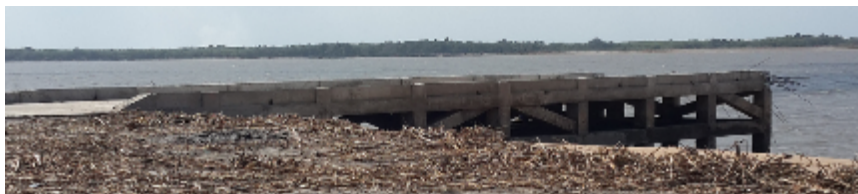
Figure 5.8. An harbour being build in Chinde.
