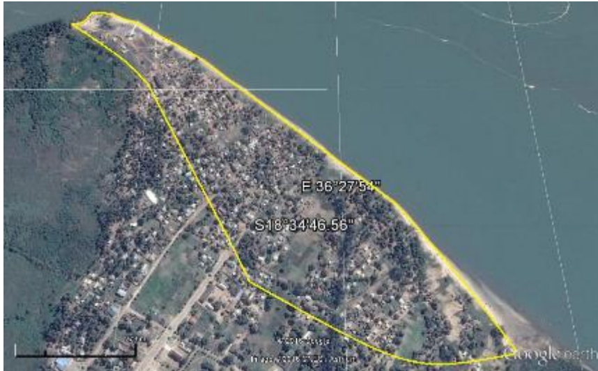
Figure 5.7. Area adjacent to Chinde Beach threatened by erosion.
