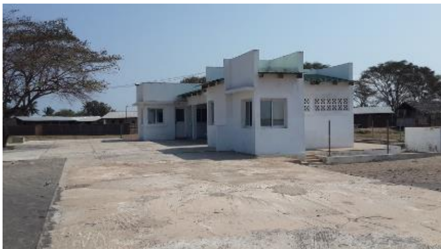
Figure 5.9. The building for maritime administration in Chinde.
